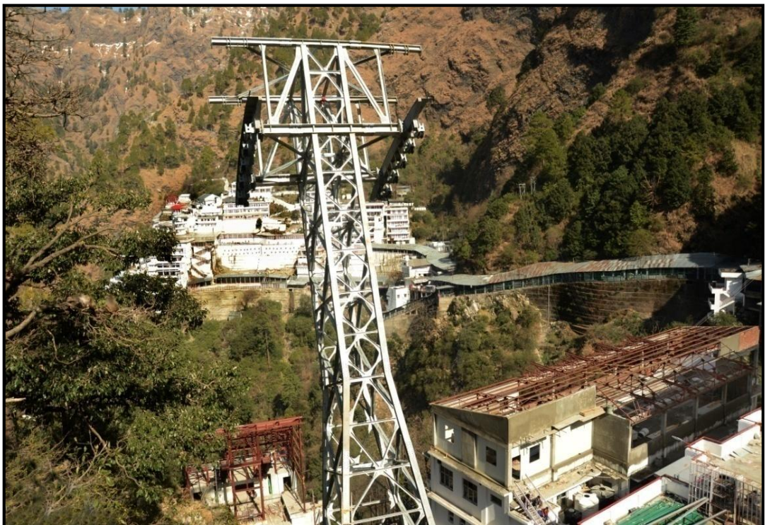
Lower tower of Bhawan-Bhairon Ghati Passenger Ropeway under installation
