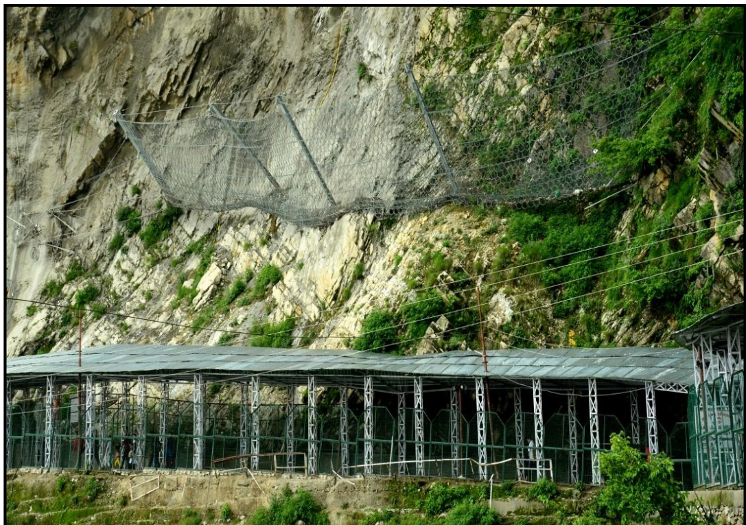
Slope Stabilisation work on Himkoti Marg
