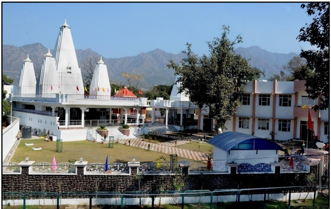
Shri N. N. Vohra, Hon'ble Chairman of the Shrine Board dedicated Renovated Mahadev Temple Complex and Yatra facilities to people at Reasi on 08-04-2016
