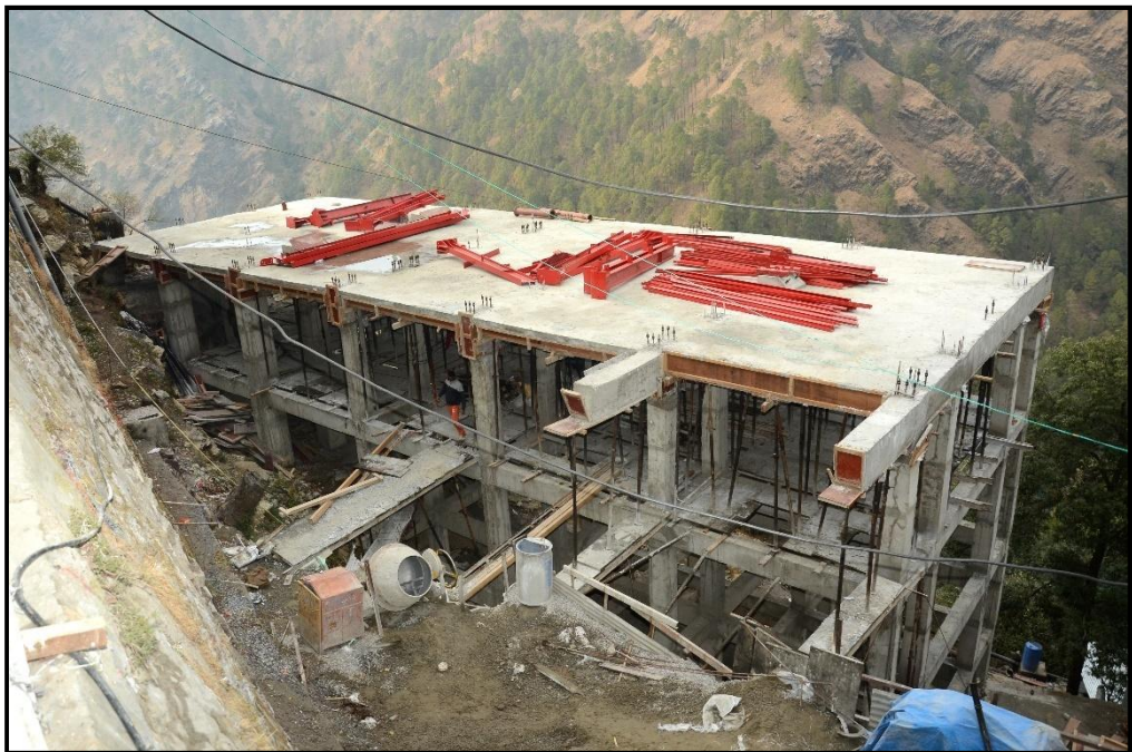
Under construction Upper Terminal of Siar Dabri-Bhawan Material Ropeway
